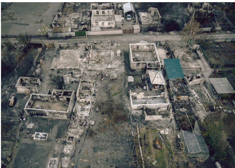
Figure 8. Destruction of residential buildings in Smolianynove village as a result of a forest fire (Photo by Oleksiy Kovaliov)
